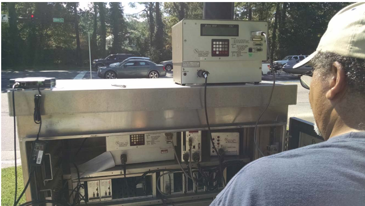
Traffic Signal Electronics Technician II Steve Smith installing a radio on site at Shore Drive/Helicopter Road.
