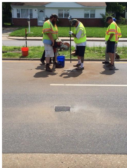
Detector installation on Virginia Beach Boulevard
