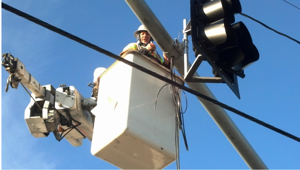
Signs & Marking Mechanic Charles Patterson bolting signal to new mast arm
