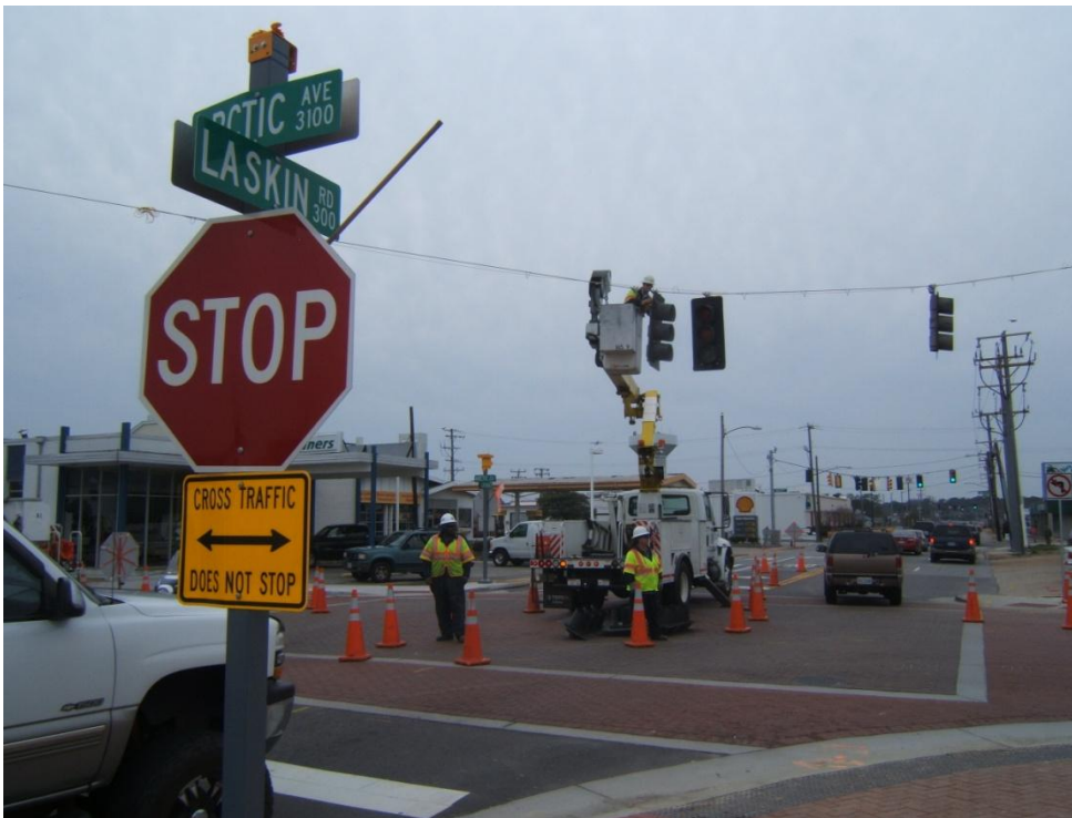
Laskin Rd and Arctic Ave temporary traffic signal installation. (Facing west)
