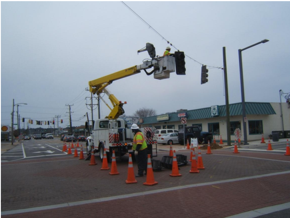
Laskin Rd and Arctic Ave temporary traffic signal installation. (Facing northwest)
