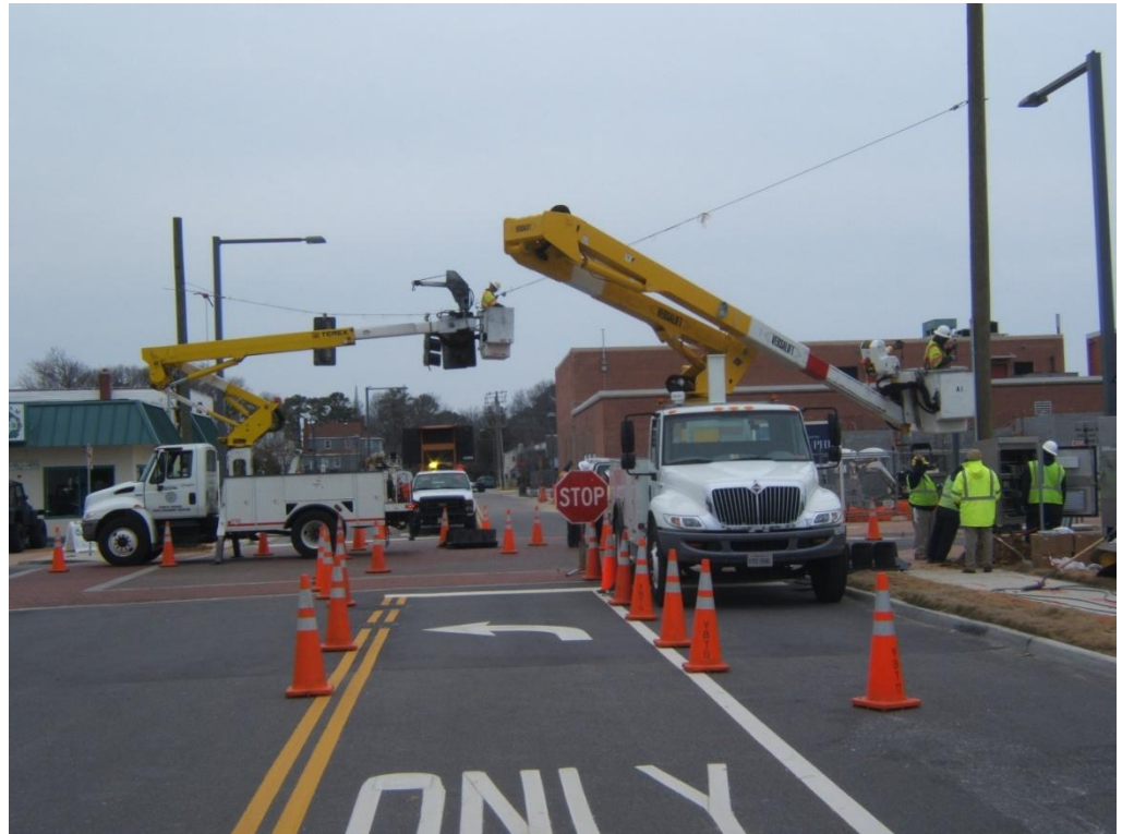
Laskin Rd and Arctic Ave temporary traffic signal installation. (Facing north)
