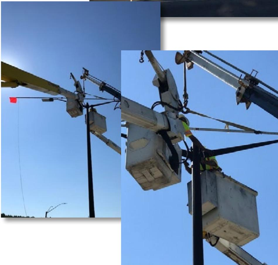
Staff reinstalling light fixtures to the new support sleeve.
