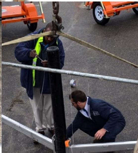
Staff designed and fabricated this support bracket. This bracket held the streetlight arms and fixtures in place in the air while the new fiberglass sleeve was installed. This allow immediate reattachment of the light fixture after the new sleeve was in place.
