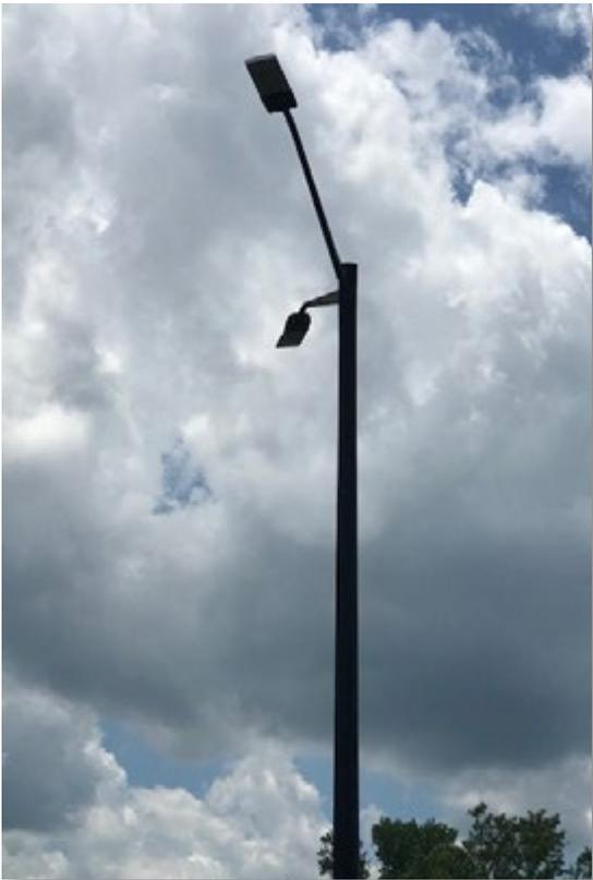
Ground level view of off-center light fixture. Light arms should be perpendicular to the pole NOT angled as shown.
