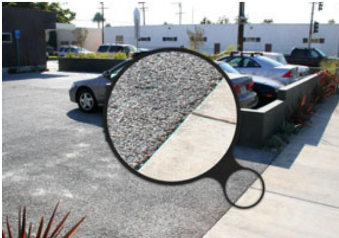
**POROUS CONCRETE:** There are a number of alternate names for porous concrete including permeable concrete, porous pavement, and pervious concrete. All of the names basically mean the same thing; porous concrete is a form of concrete which is permeable, rather than solid. Porous concrete is designed to trap water and allow it to percolate through the concrete to the ground below. Pervious concrete uses the same materials as conventional concrete, with the
