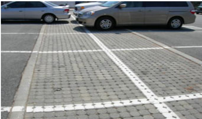
**OPEN JOINTED AND OPEN CELL PAVING BLOCKS:** These pavers are solid units of concrete, brick, plastic or stone laid side by side. They can bear traffic loads and are shaped to produce openings that are filled with porous aggregate or turf that allows for infiltration of stormwater.
