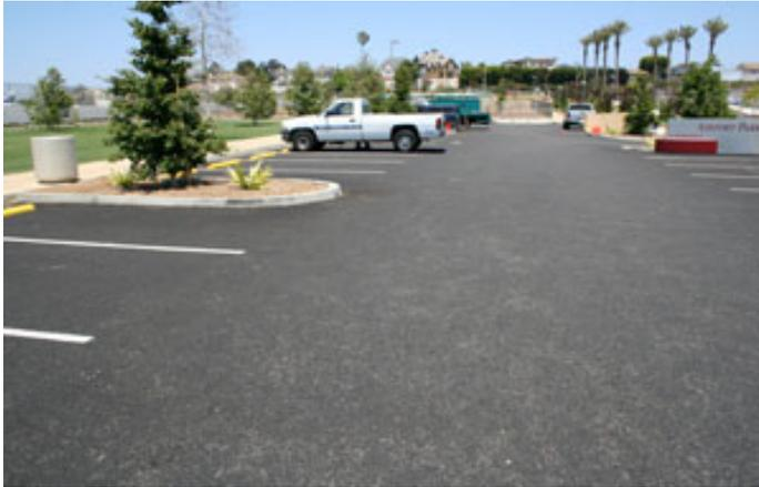
The water drains through the porous asphalt and into the stone bed, then, slowly, infiltrates into the soil. If contaminants were on the surface at the time of the storm, they are swept along with the rainfall through the stone bed. From there they infiltrate into the sub-base so that they are subjected to the natural processes that cleanse water.
