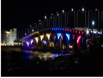
Lesner Bridge lighting
