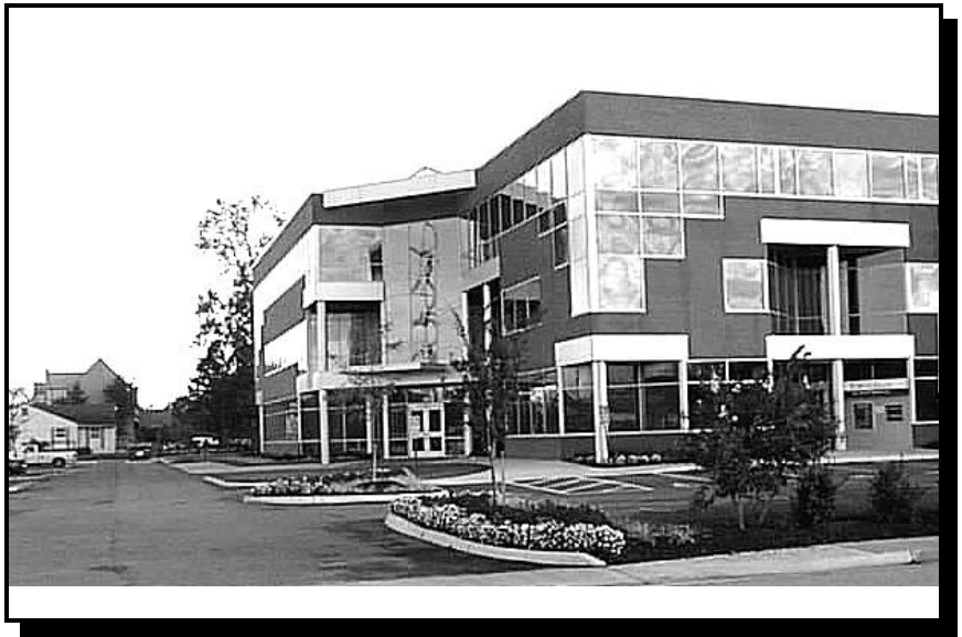
A well maintained office building with good visibility around the entire perimeter.
