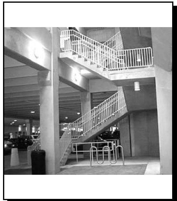
This open stair provides good visibility from store entrance as well as the parking area.
