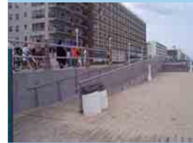
8th Street handicap access ramp and timber walkway
