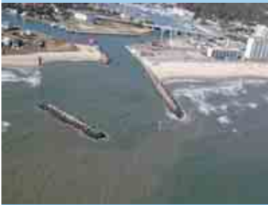
Rudee Inlet jetty system
