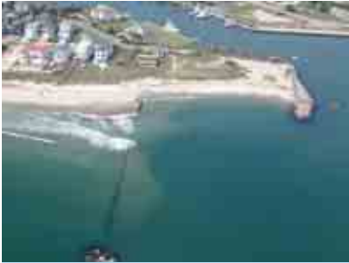
Rudee Inlet's aging timber weir and southern jetties
