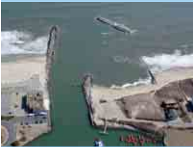
Rudee Inlet Jetty System
