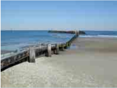
Rudee Inlet timber weir
