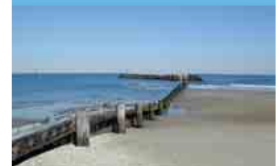
Rudee Inlet Timber Weir
