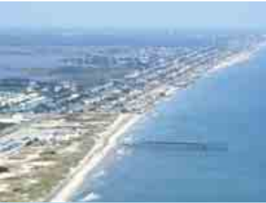
Effects of erosion at the South End - August 2001
