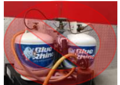
Regulator not at tanks
